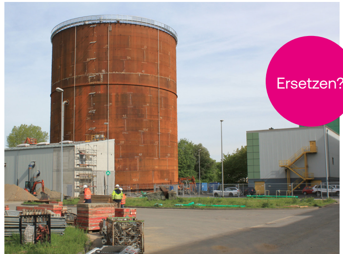
District heating storage facility (construction phase) for increasing the proportion of CHP.
